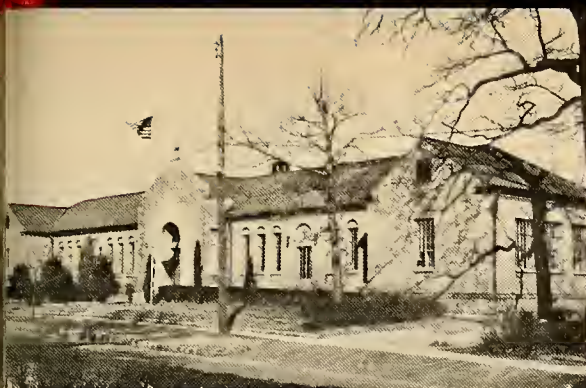
Front view of school and entrance to church
