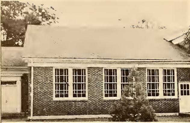
A corner view of classroom building
