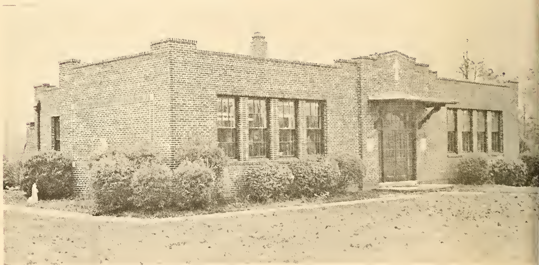
View of classrooms
