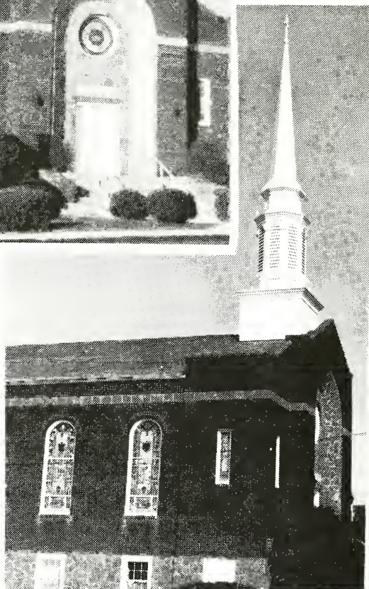
After Installing Steeple — 1983
