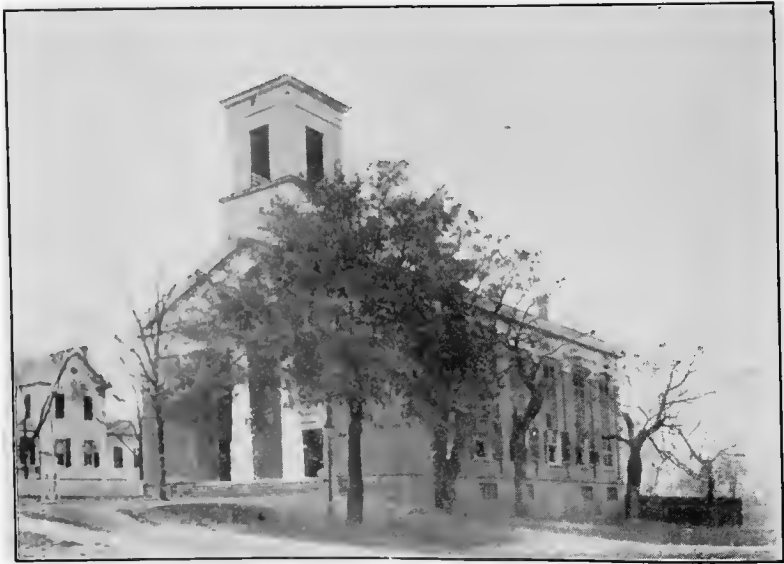
MULBERRY ST. METHODIST CHURCH, BEFORE REMODELLED.
