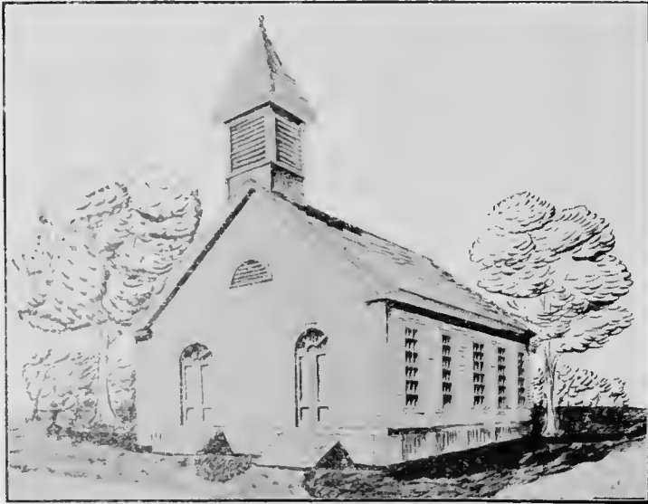
METHODIST CHURCH, 1828. FIRST EVER BUILT IN MACON.
