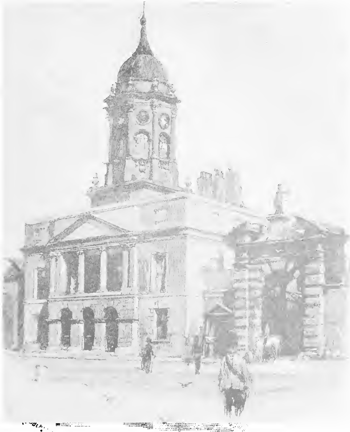
(THE CLOCK TOWER, DUBLIN CASTLE.)
