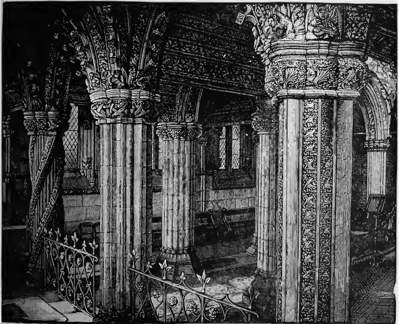
(INTERIOR OF ROSLYN CHAPEL, from a photograph by G. W. Wilson & Co.)
