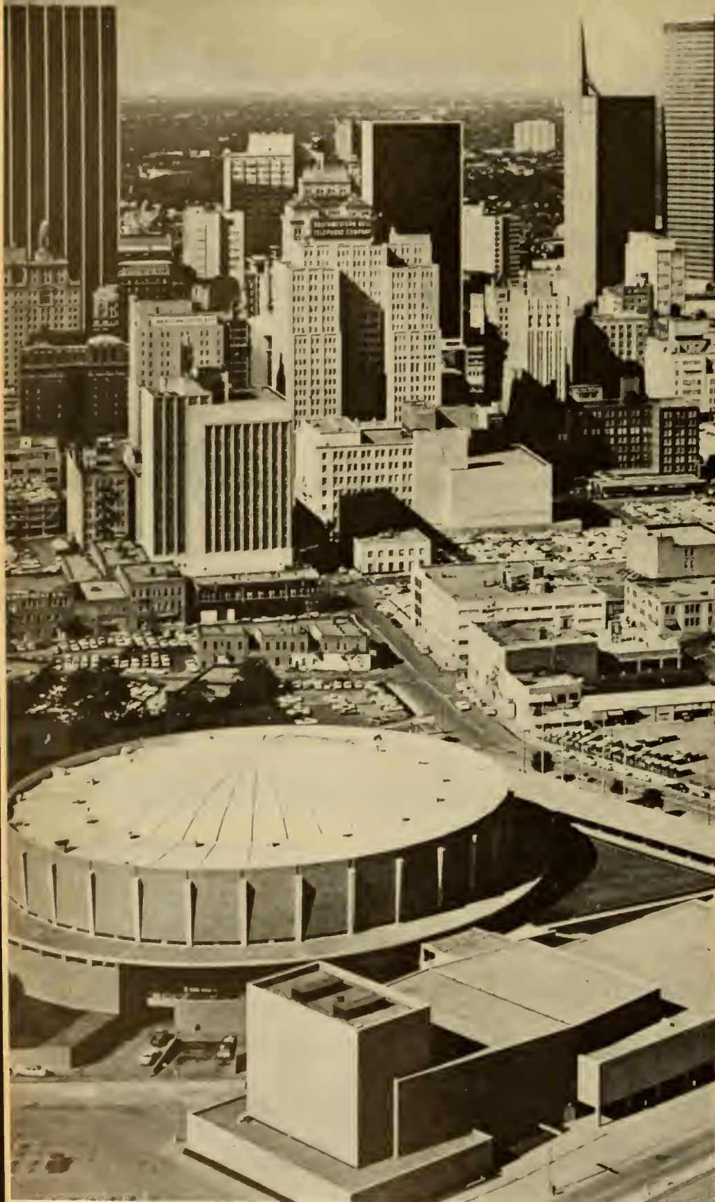
Dallas Memorial Auditorium, the mammoth circular building in the foreground above, will be the site of the 1968 Uniting Conference of The United Methodist Church, bringing together Methodists and Evangelical United Brethren into a new 11-million member church. Rising beyond the auditorium are the sleek skyscrapers of downtown Dallas.
