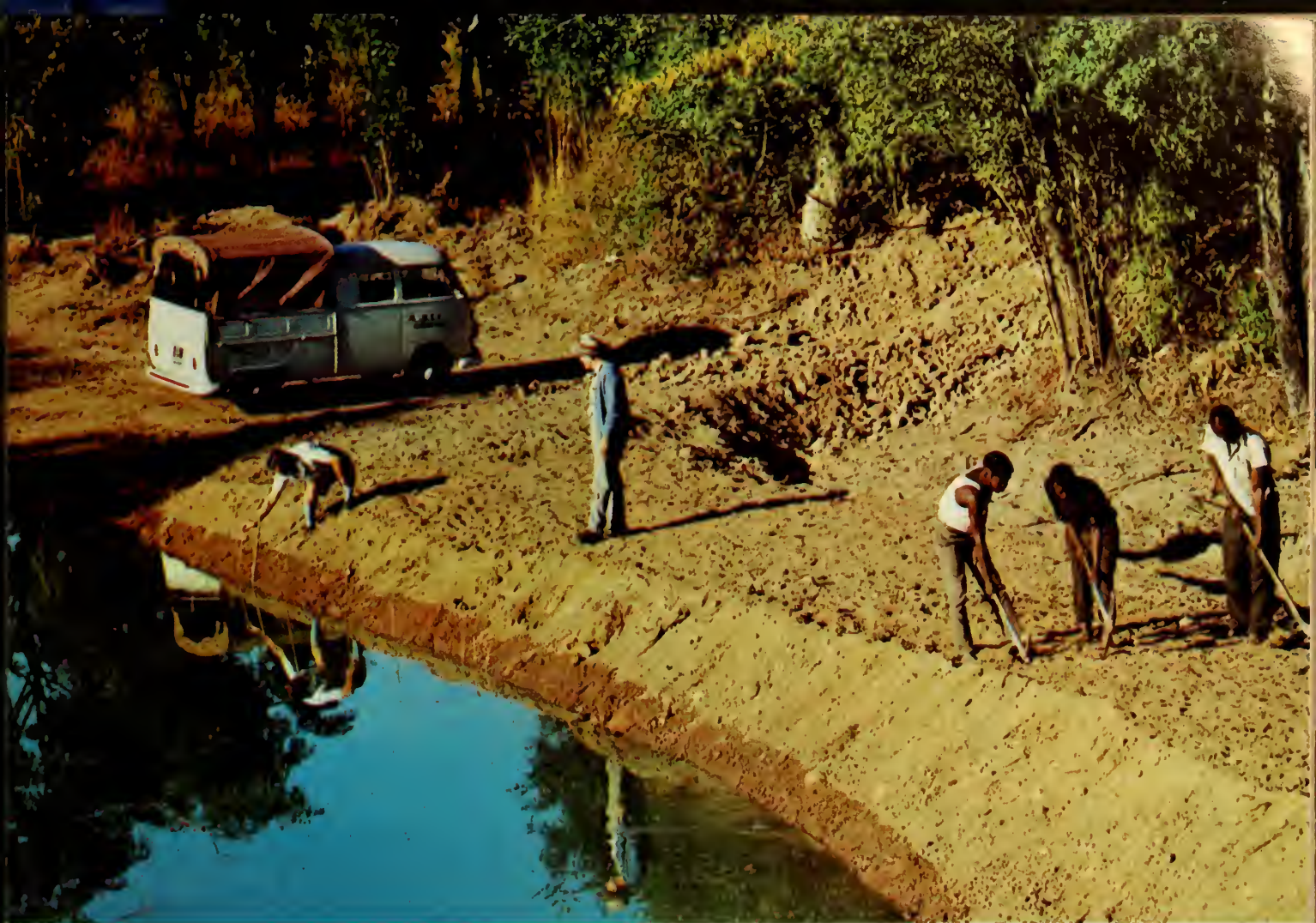
Trainees turn up an earthen dam to hold back water for an irrigation project. Although rainfall is said to be adequate, it may arrive during the wrong season, and can be destructive. Many amateur farmers fail in the Copperbelt area where soil is poor and bush-clearing costs are high.
