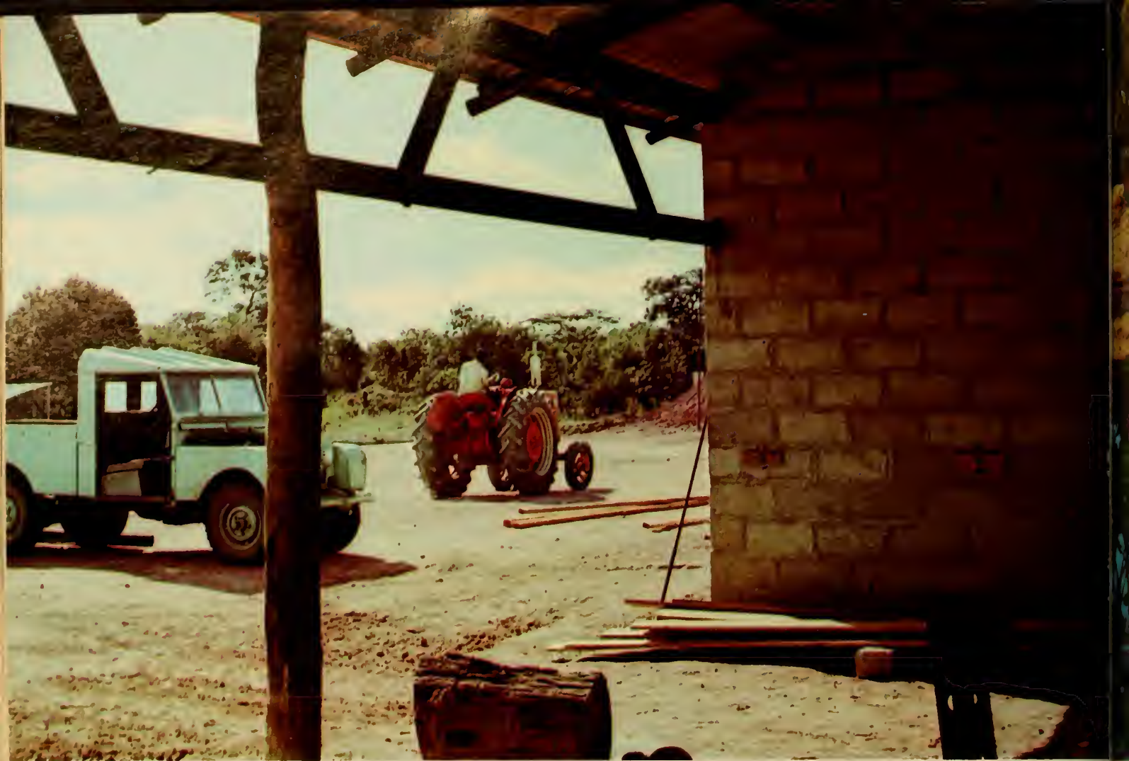
One of the most important buildings at the Mindolo training center, as on any large farm, is the machine shed and shop. Here it is that young Zambians, who will operate their own farms after graduation, learn how to care for tractors and other agricultural equipment.
