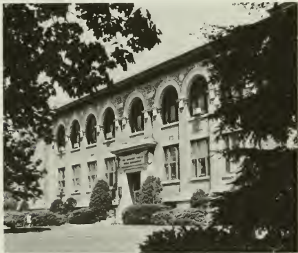
FREE METHODIST CHURCH HEADQUARTERS, WINONA LAKE, INDIANA
