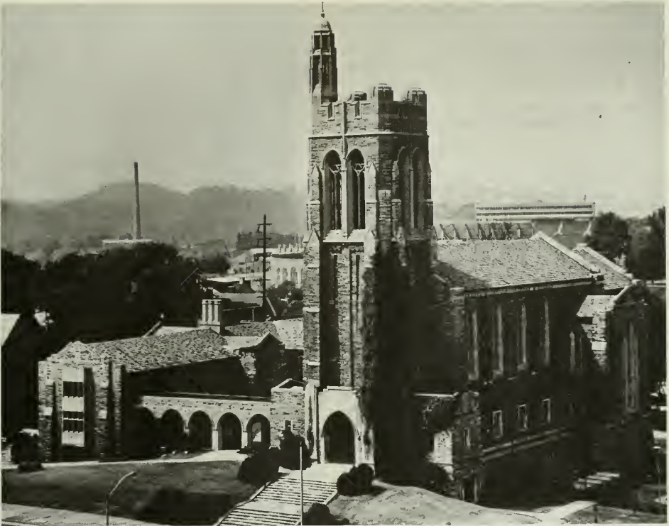
CHURCH STREET CHURCH, KNOXVILLE, TENNESSEE
