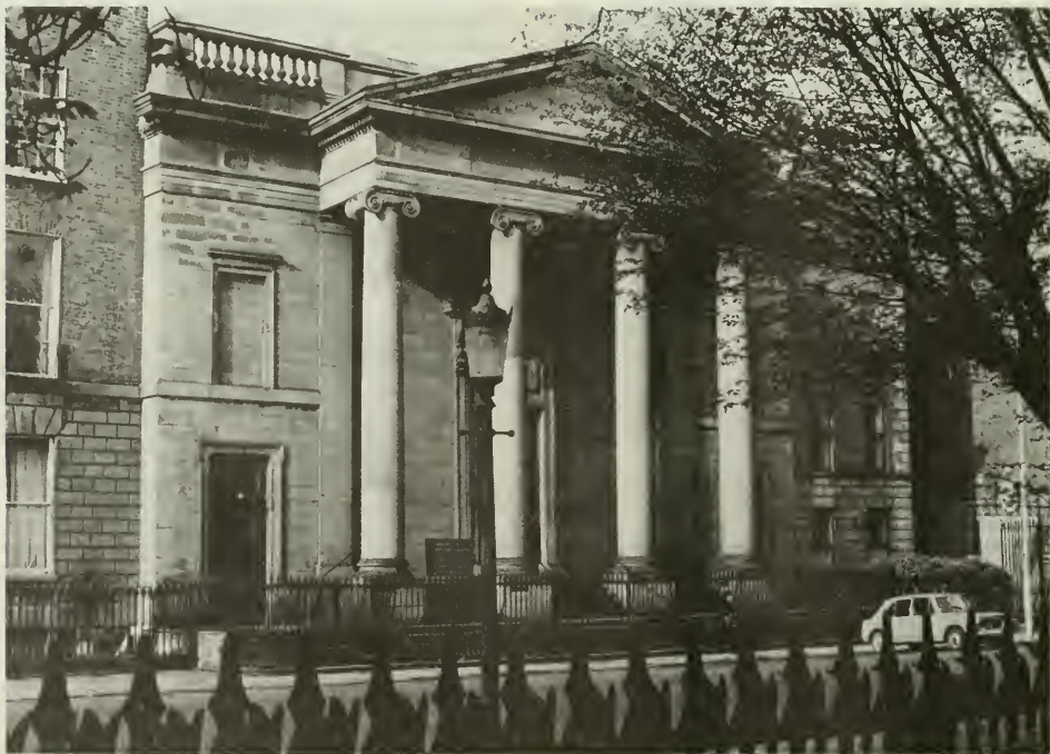
CENTENARY CHURCH, ST. STEPHEN'S GREEN, DUBLIN, IRELAND
