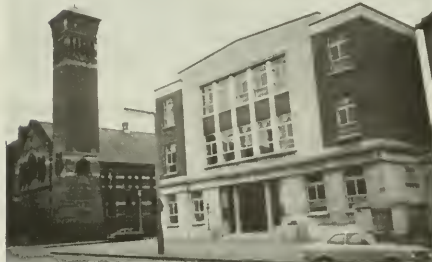
ALDERSGATE HOUSE, BELFAST
