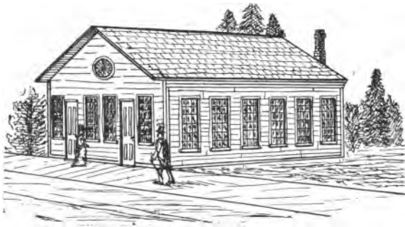
FIRST METHODIST CHURCH, TORONTO, ON SITE OF PRESENT BANK OF COMMERCE, COR. KING AND JORDAN STREETS.
