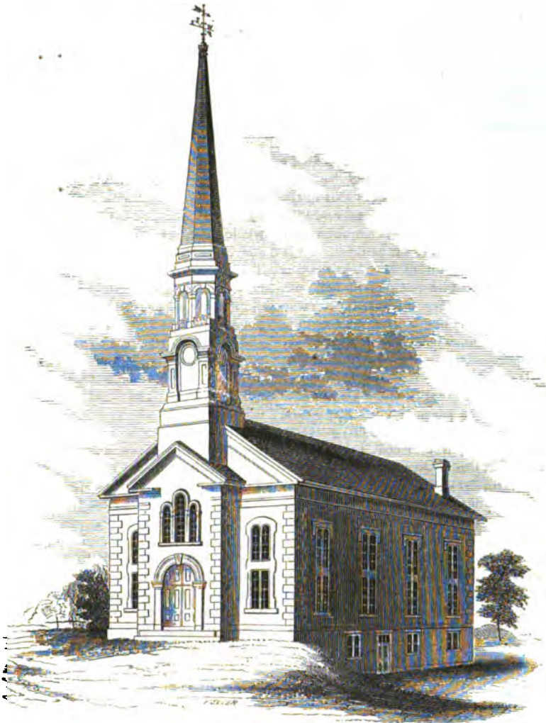
BEACON-STREET METHODIST EPISCOPAL CHURCH, BATH, ME.
