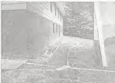
A new sidewalk has been poured behind the Mattie Parsons Building
