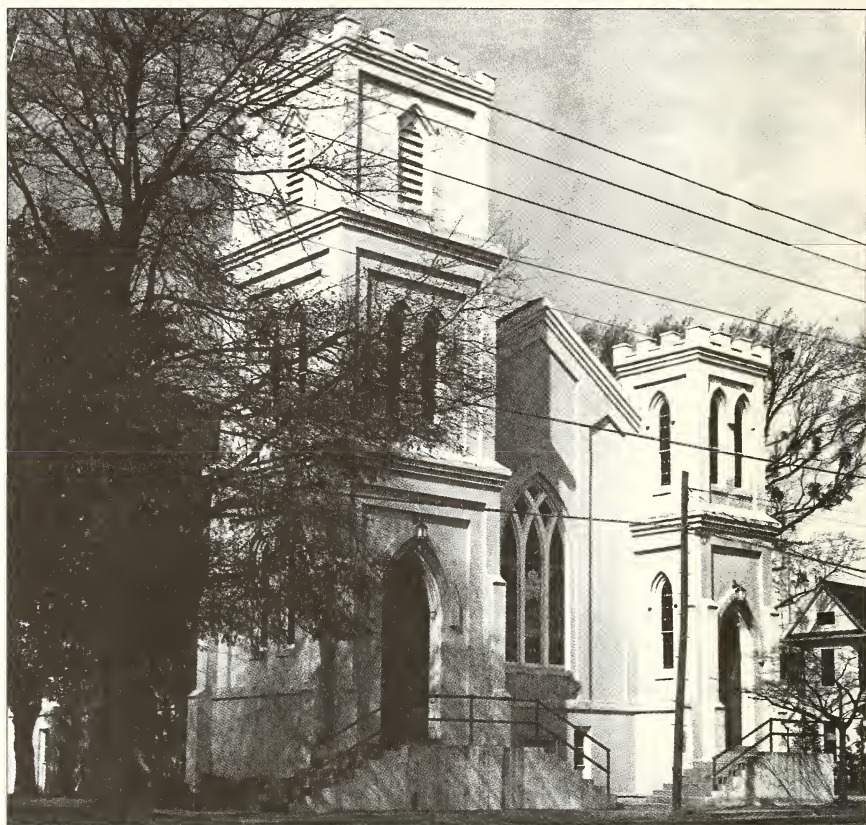
Front view of The Memorial Baptist Church, Fourth and Greene Streets after addition of the tower. (Courtesy of the Daily Reflector).
