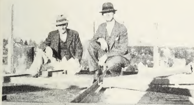
Elder A.A. Cashion, construction superintendent, and Rev. Watt M. Cooper, on top of the spire platform, December 1948.
