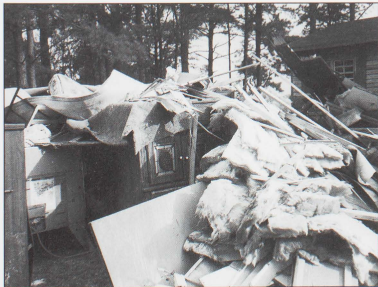
Carpeting, insulation, appliances, beds, and furniture piled high outside this home reveal the devastation from flood waters following Hurricane Floyd.
