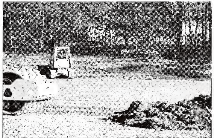
Work on the New Gym has begun.
