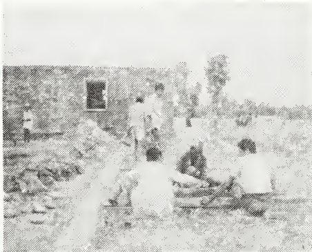
Construction of school building in Olani, Nepal.
