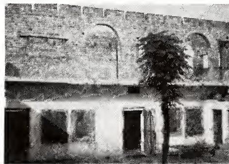
Moga Church under construction in State of Punjab.
