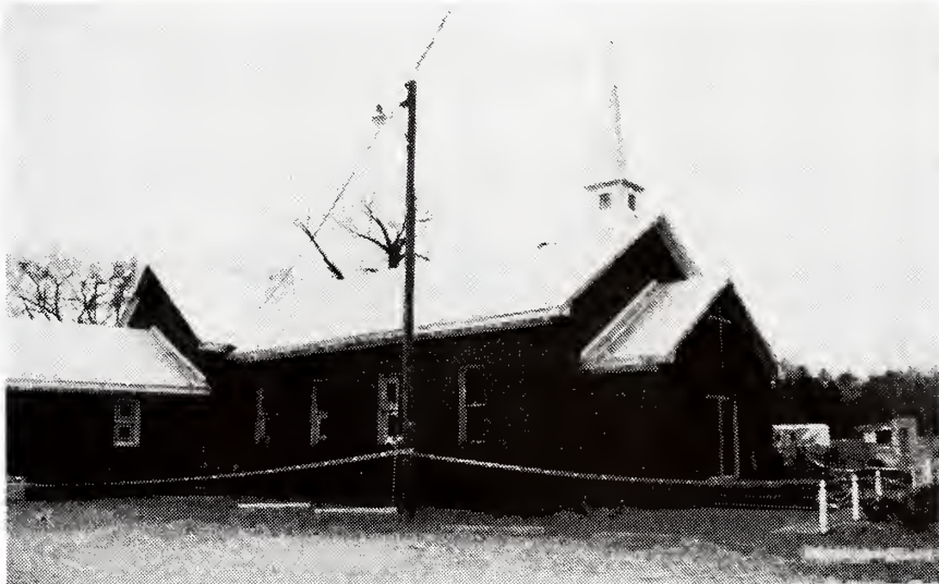
Broken windows and smoke damage bear witness to the charred interior of the church.
