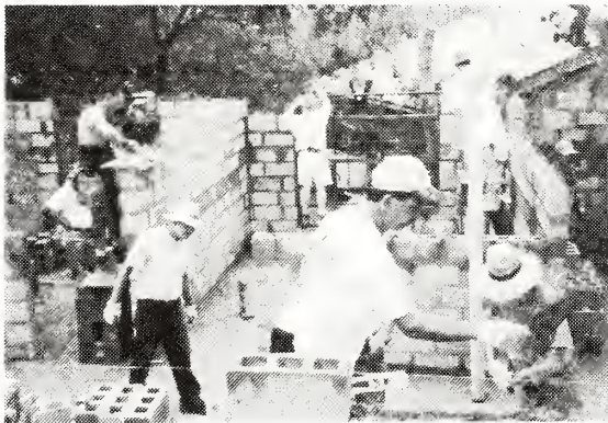
Walls almost complete on Tuesday afternoon
