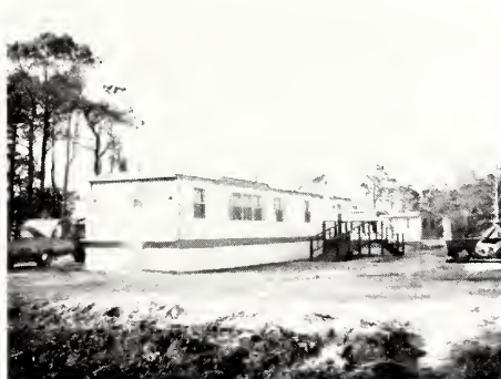
Vinyl skirting installed on the mobile church.
