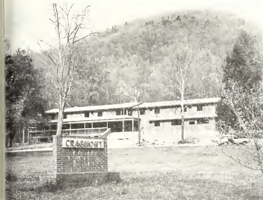
New building at Cragmont
