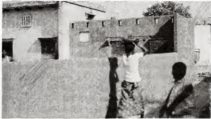
Construction at Satpur
