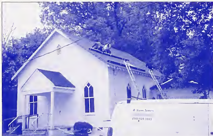
Windsor Church gets a new roof!
