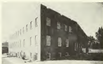
EDUCATIONAL BUILDING - ERECTED 1939 - Rear View
