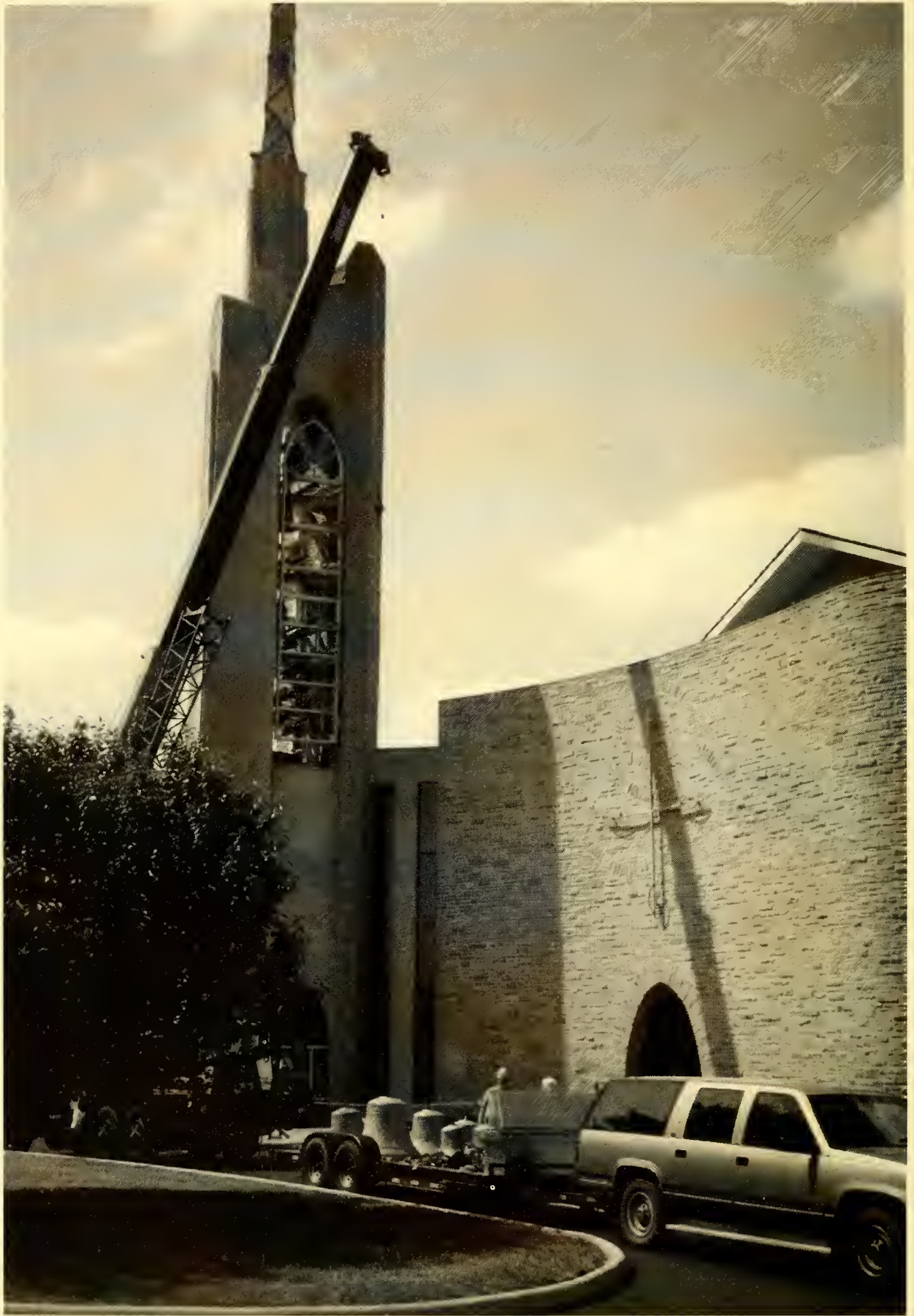
Refurbishing of carillon bells, summer 2002.
