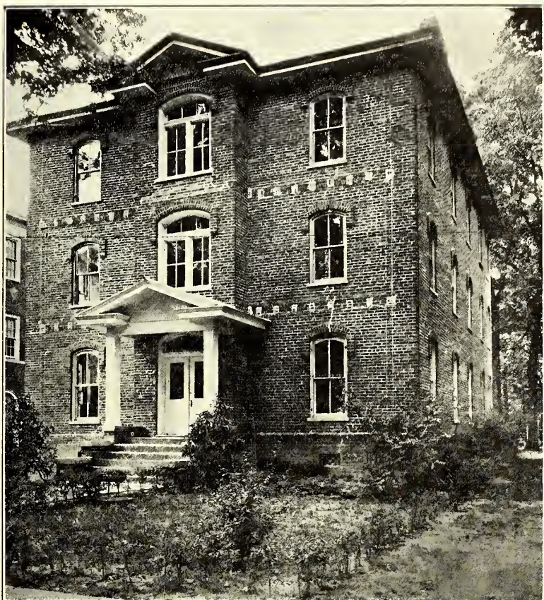
EAST DORMITORY IS THE OLDEST BUILDING ON THE CAMPUS, YET ONE OF THE MOST MODERN DORMITORIES.
