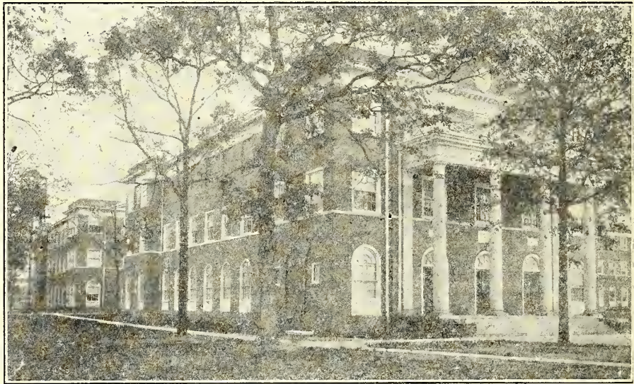
Whitley Memorial Auditorium Building, Elon College, housing the chapel and Music Department.
