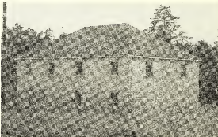
ZION'S NEW EDUCATIONAL BUILDING
