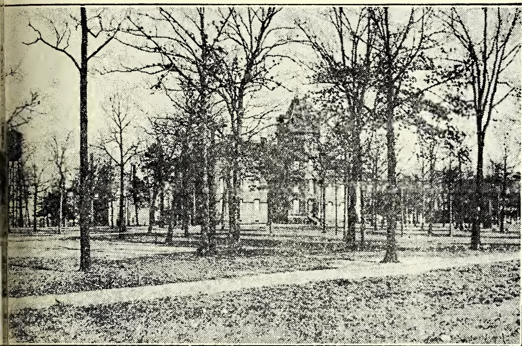
ANK POWER HOUSE ADMINISTRATION BUILDING FACING THE WEST DORMITORY
