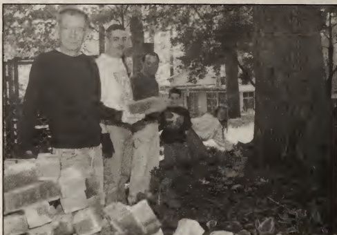
Lending a helping hand... Members of the St. Gabriel Parish Men's Club and the St. John Neumann Knights of Columbus Council #7343 recently pitched in after a brick wall collapsed in the backyard of the bishop's residence in Charlotte's Dilworth neighborhood. Pictured from left are Knights John G. Sell, John A. Sell, and Mike Horeth with Jordan and Madison Horeth.
