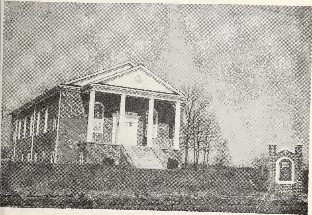
BUILDING AT DUNCAN, S. C.
