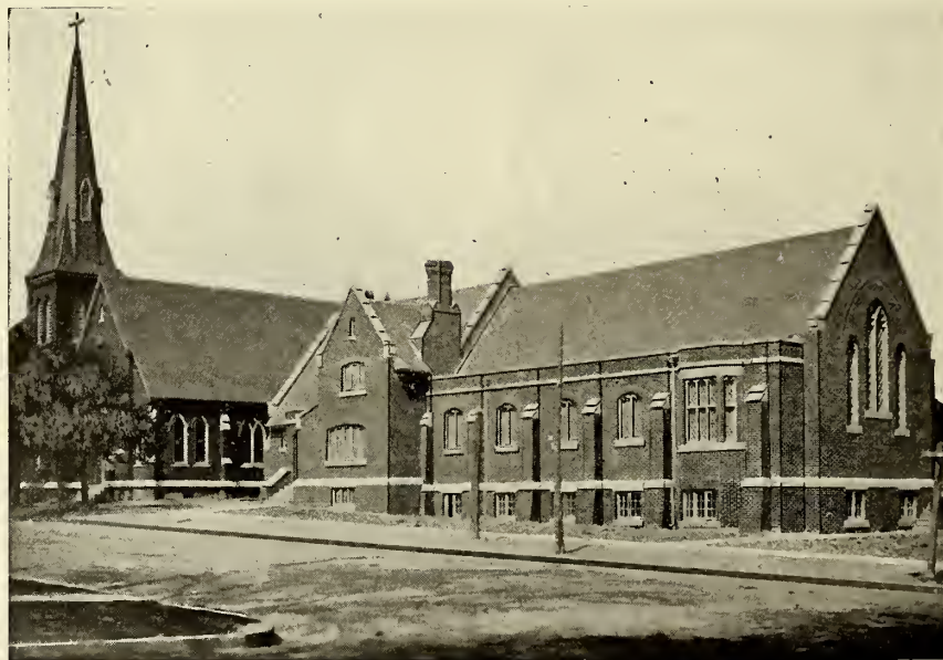
THE CHURCH AND NEW PARISH HOUSE AT HENDERSON
