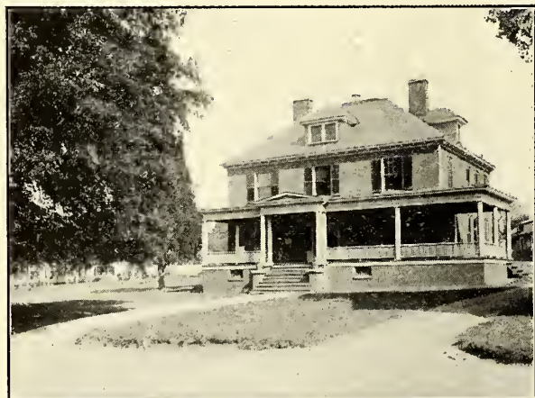
THE STEDMAN MEMORIAL BUILDING—THE SUPERINTENDENT'S HOME
