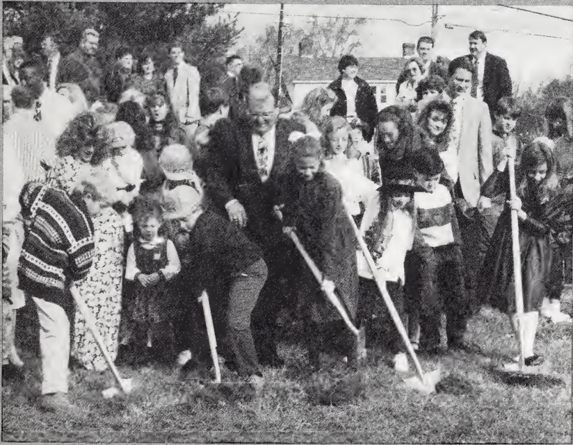
Ground Breaking Friendly Avenue Church of Christ, Greensboro, NC See Story on Page 14
