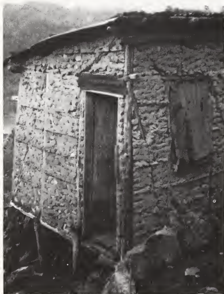
Jamaican house with repaired roof.
