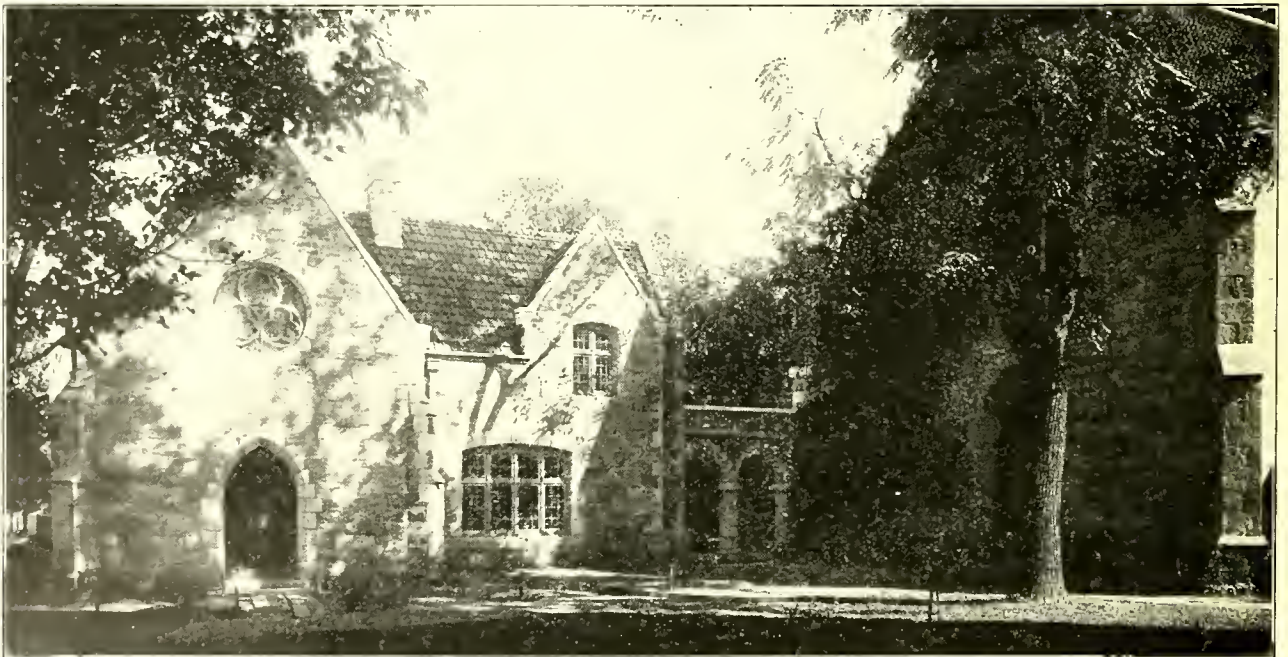
PARISH HOUSE, CHRIST CHURCH, RALEIGH (View from Capitol Square, Northeast)
