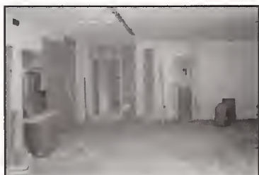
Nelson Home prior to renovations.
