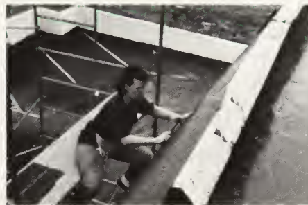
Miriam nailing on shingles
