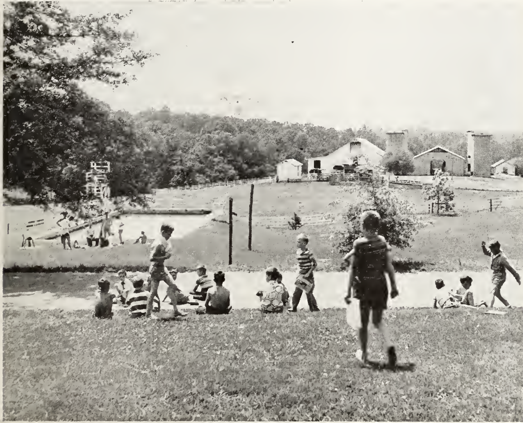
The most interesting spot on the campus during the summer days is the swimming pool. Although it leaks badly and can be used only part time, the boys and girls love to cool off in it.
