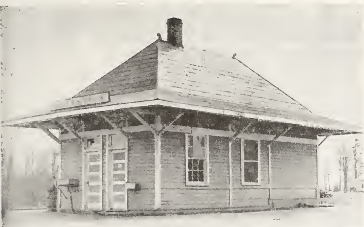
Barium Depot and Post Office, one of the oldest remaining landmarks at Barium to be moved.
