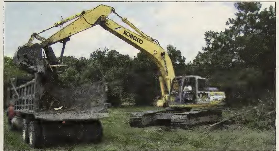
Global Construction completing site preparation on lots #9 & 10.
