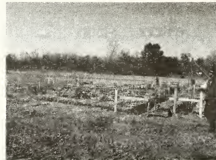
At left, foundation is dug for first home site.
