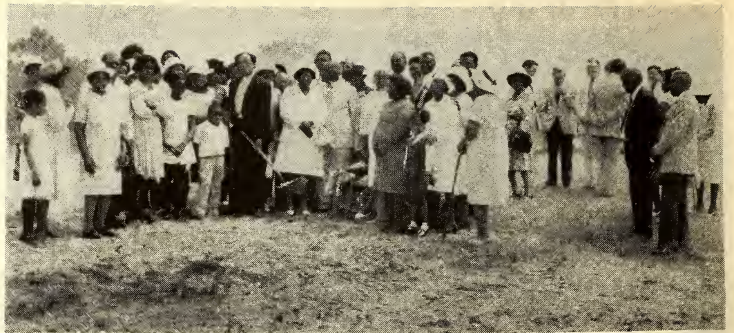
Members of Cherry Chapel Baptist Church, Hobgood, at their ground breaking service, Sunday, June 4. Rev. S.J. Jones, Pastor is shown with shovel.
