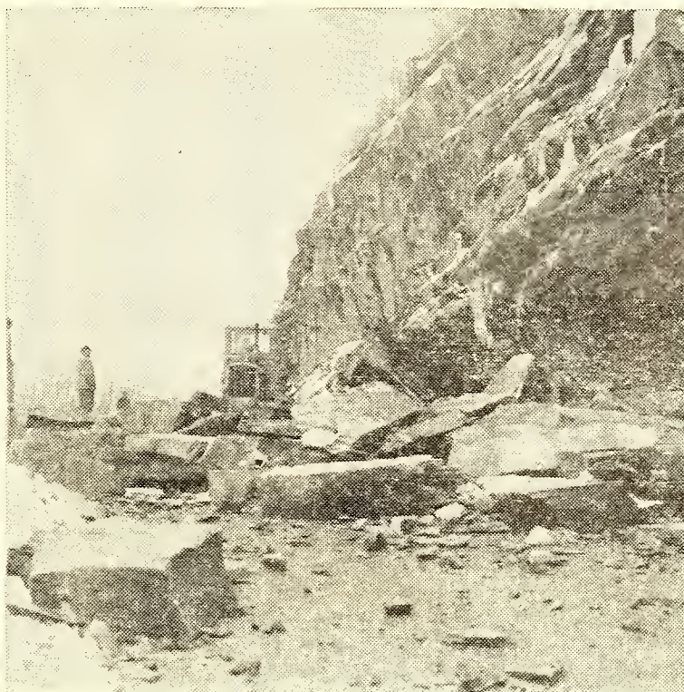
ROCKS THAT FALL INTO THE ROAD at the Jumping Off Place on the main road, No. 16 that comes into Ashe county.
