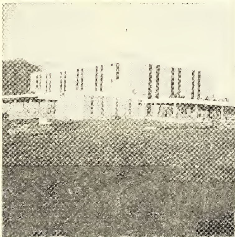
NEW ASHE MEMORIAL HOSPITAL was dedicated on October 30.
