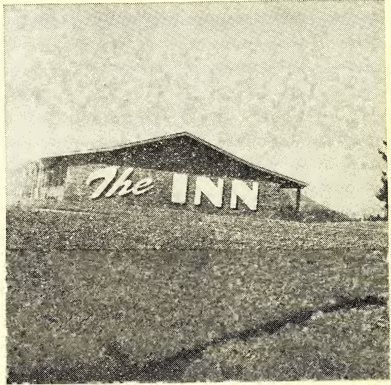
THE INN, the new motel which has just been built at Glendale Springs.
