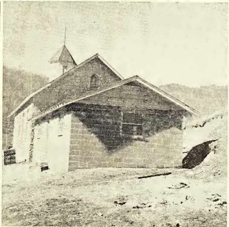
NEW SUNDAY SCHOOL BUILDING at Bethel-Millers church in Wilkes county was built by members of the church and the money raised by them.
