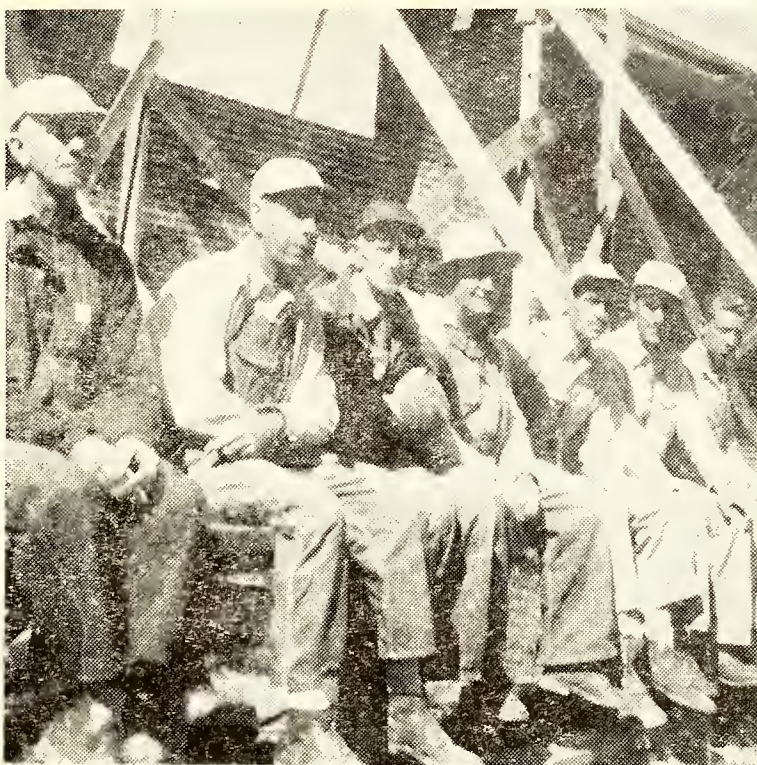
MEN WHO HAVE WORKED ON MEMORIAL building are these who work with well known contractor, Bert Dixon.
