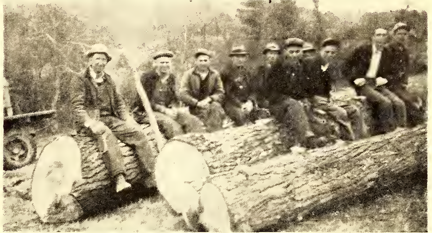
Part of the volunteer workers are shown on logs to be used in Ebenezer Presbyterian church that is now under construction.
