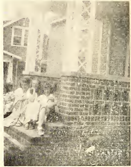
New porch built to the Lansing manse. The building of the porch was supervised by Elder J. O. Blevins.
