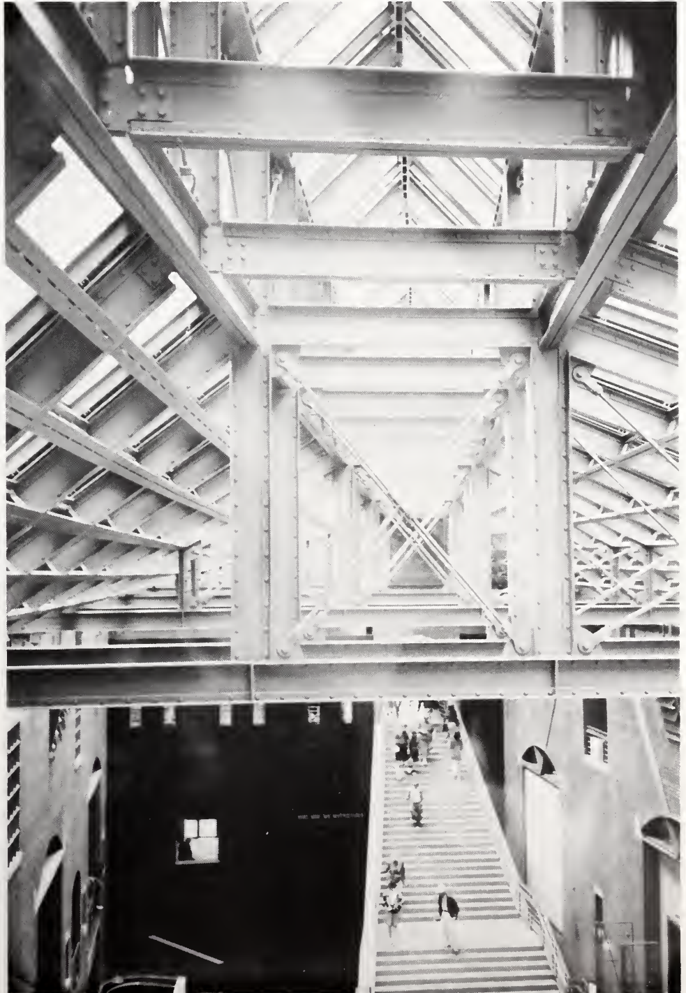
Grand staircase and exposed steel beams in the Hall of Witness, central gathering place of US Holocaust Memorial Museum.
