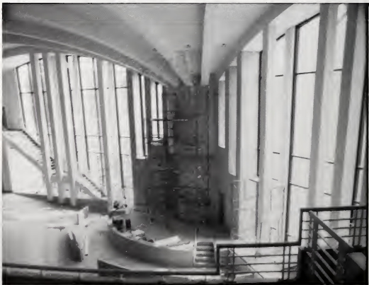
Work in process on the interior of the sanctuary.
