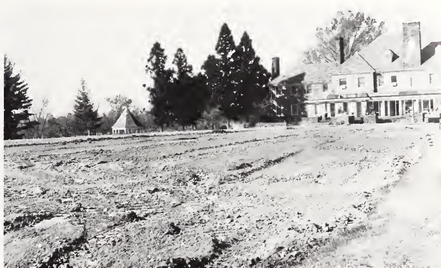
A view of the Home as it appeared ready for the dream to continue to build.
