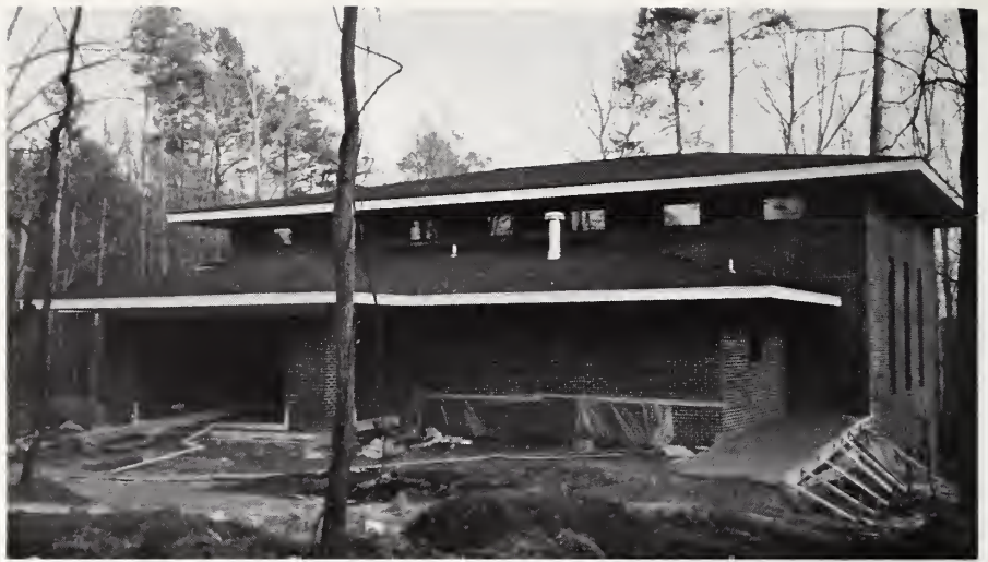
Beth Shalom Synagogue under construction.
