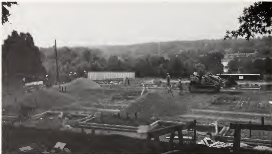
Above: The outline of the Personal Care Unit takes shape.
