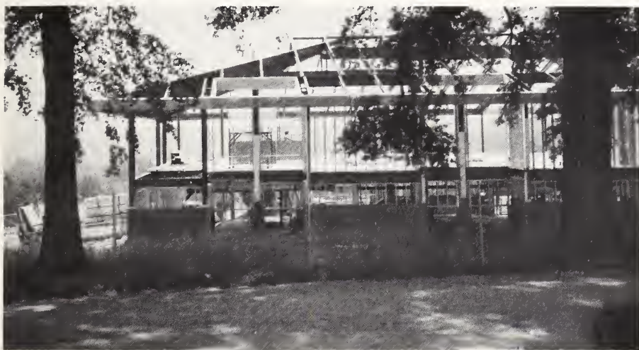
Above: FAIR OAKS before the brick and shingles went on. Right: Uppermost section of Commons is framed in. This creates a 30' ceiling in the lounge and entry!
