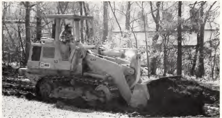
Sign of the times – earthmoving equipment. Here, the workman grades for a new parking lot.
