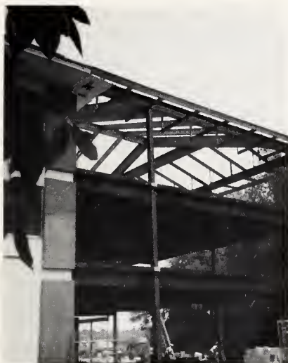
B-Wing expansion will house new dining rooms, pantries, and elevators.
