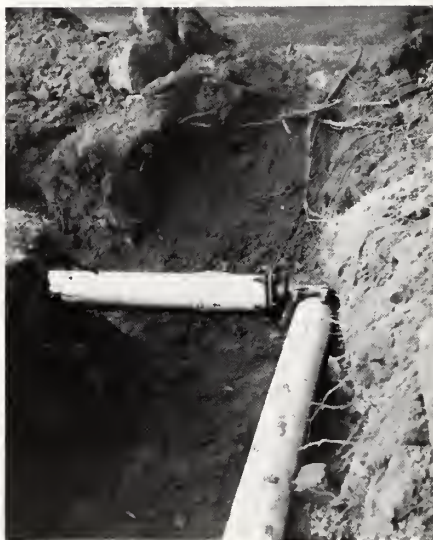
At Right: Water lines encircle the property to assure supply to the fire sprinkler system.
