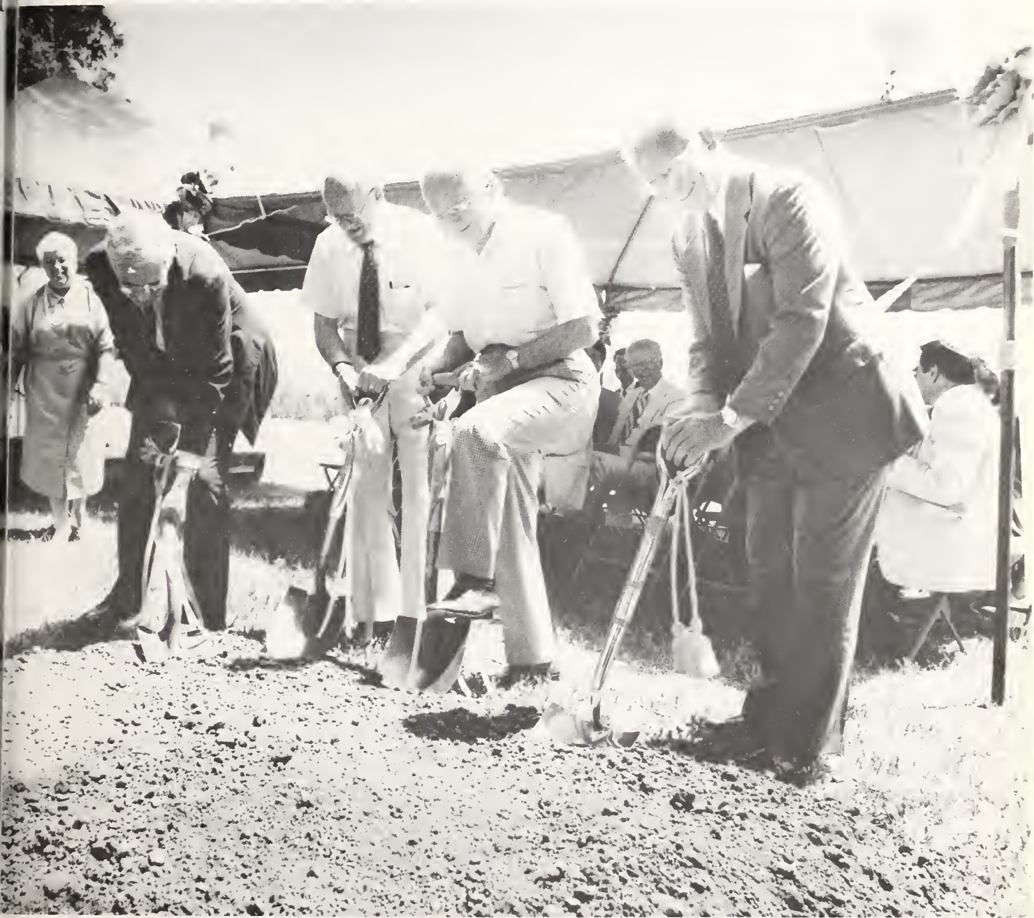
Groundbreaking at Blumenthal Jewish Home—Story on Page 23
