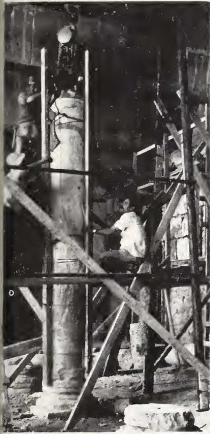
Toppled pillars being returned to their original positions on the Cardo, an ancient Roman street now being restored in Jerusalem.
