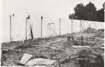
Construction begins for the 3-floor B Wing, 1974.
