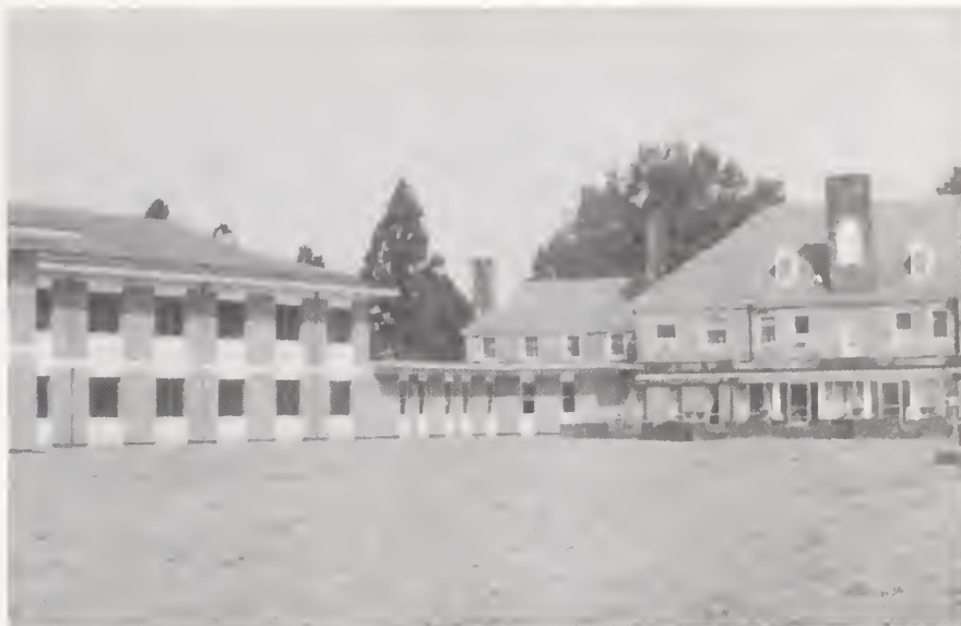
Looking east towards the new wing (left) and the mansion (right).
