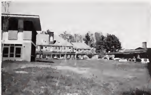
A worms eye view of the new grounds.
