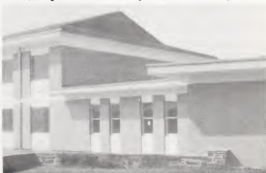
A frontal view of the portion of the new wing which connects to the mansion.
