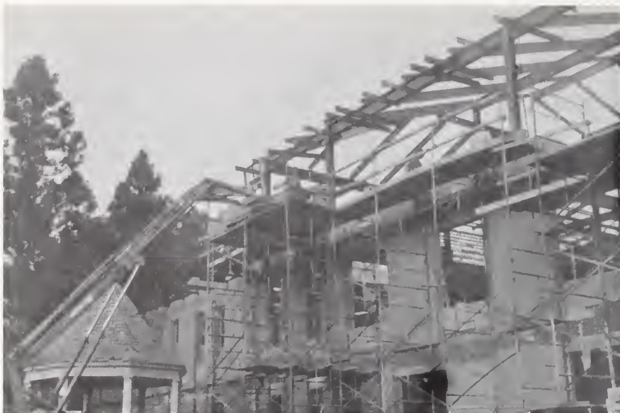
The new structure — brick and steel are beginning to take shape.
