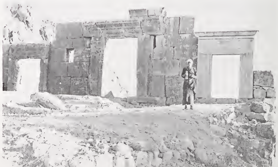
A Druze laborer stands in front of the synagogue facade in Meiron. This facade has been uncovered since antiquity. Current estimates place the building date in the 3rd or 4th centuries.
